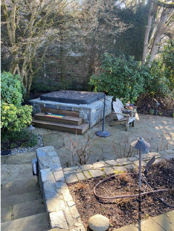
Figure 1: Existing hot tub structure to be modified.
